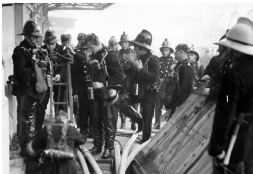
Smithfield Market fire ; point of entry and exit for the underground smoke logged areas. Photo copyright LFB /Mary Evans)
