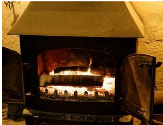
WOOD BURNERS known to produce a lot of tarry soot requiring chimney swept frequently.
